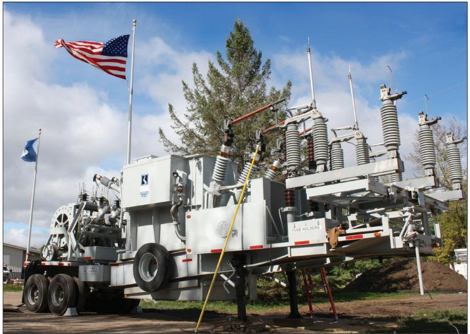
Joe continues, “The unit was installed on a Friday and powered up the following Monday. Essentially, we de-energized the line feeding into the permanent Isle sub, then set a temporary pole to feed the mobile unit. Next, we energized the mobile sub and shut down the substation.”
